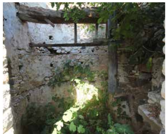
Fig. 10: Ekinlik Windmill 3, interior view and the staircase
