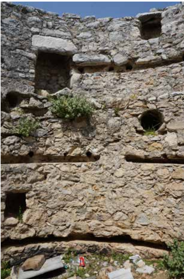
Fig. 5: Saraylar Northern Windmill, interior view
