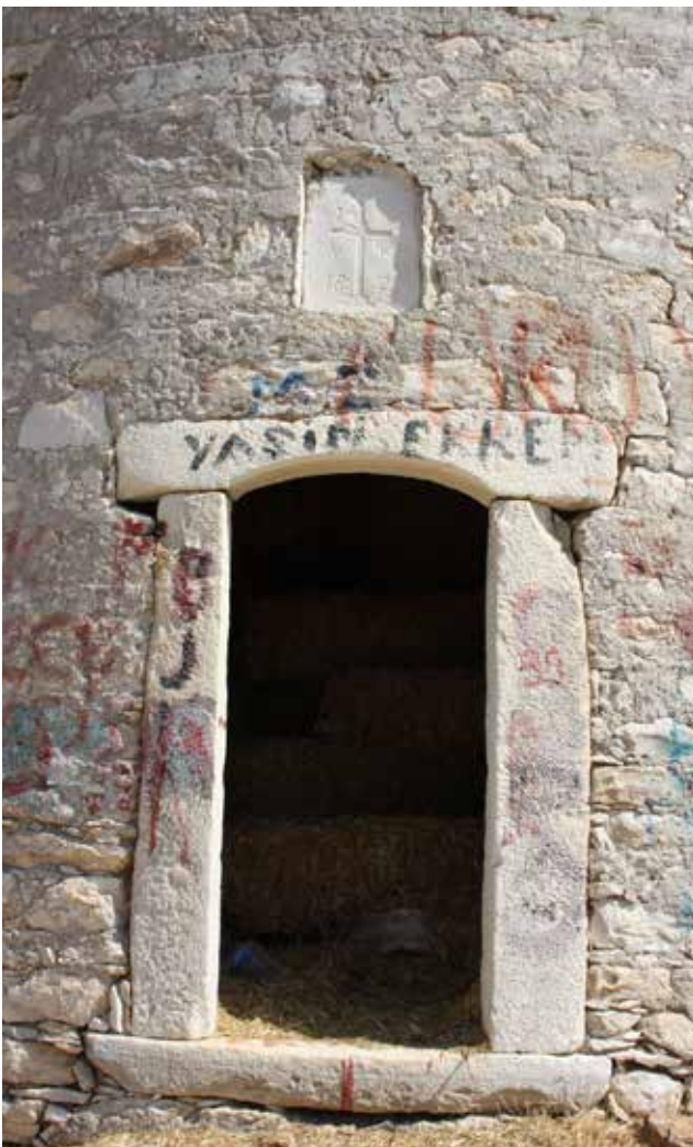
Fig. 8: Ekinlik Windmill 2, entrance door, inscription panel, and vandalism
