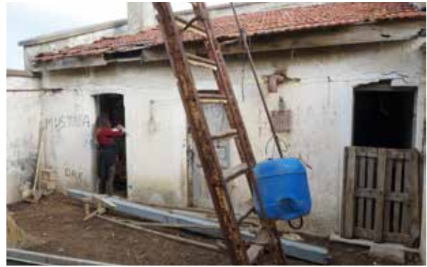
Fig. 5: Courtyard, northeastern façade
