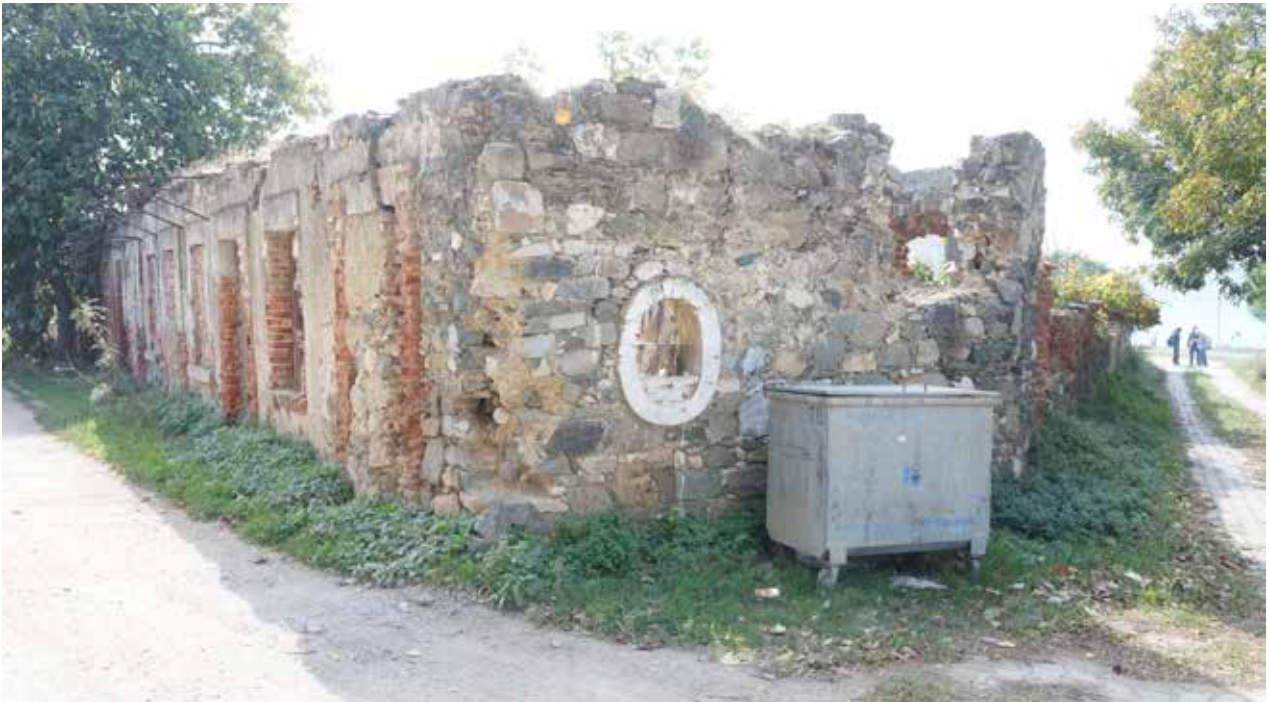
Fig. 10: Northern corner of the lodging building
