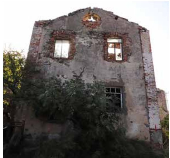
Fig. 7: Northern façade of the administrative building
