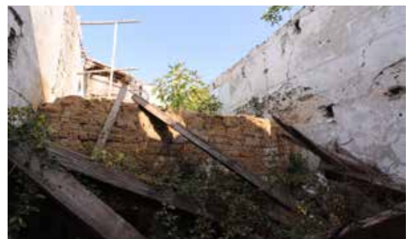
Fig. 8: View towards the north from the interior of the administrative building
