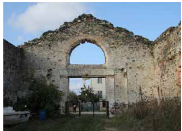
Fig. 5: Western wall of the production building
