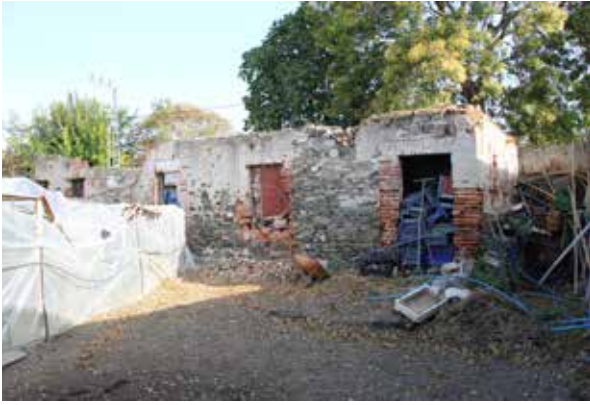
Fig. 11: Western façade of the lodging building
