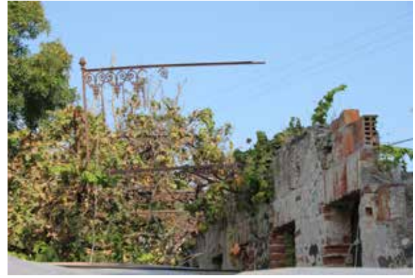
Fig. 12: Balcony railing on the western façade of the lodging building
