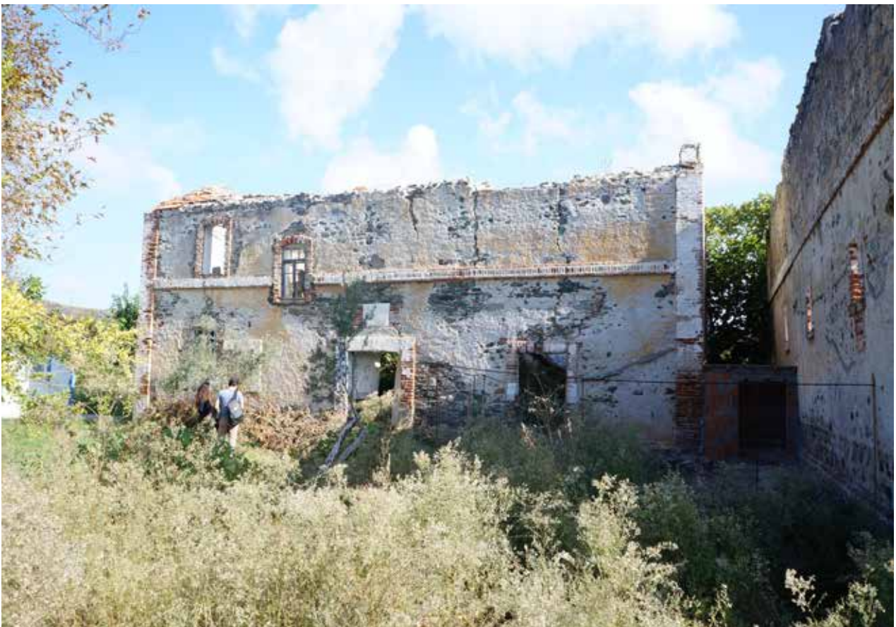
Fig. 6: Western façade of the administrative building
