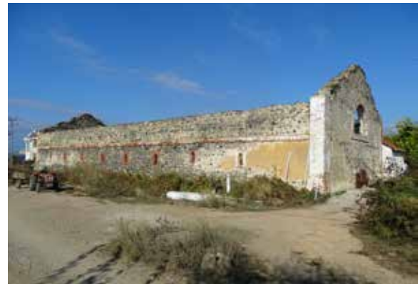
Fig. 4: The eastern and southern façades of the production building
