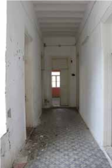
Fig. 3: Ground floor corridor with concrete tile flooring and jack-arch ceiling
