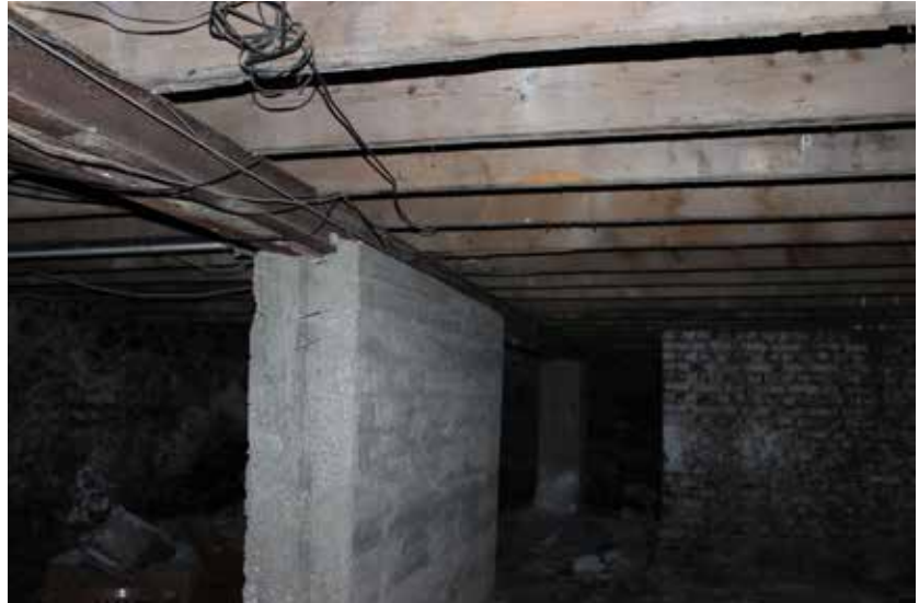
Fig. 4: Basement, reinforced concrete intervention
