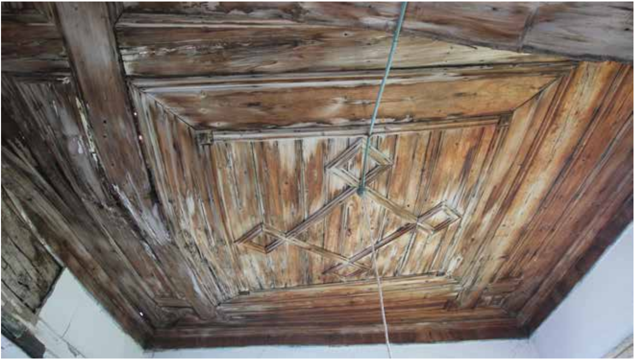
Fig. 4: Ornamented ceiling on the second floor
