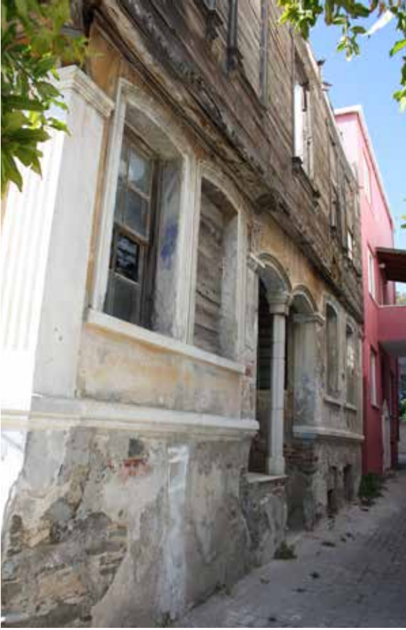
Fig. 3: Eastern façade, general view
