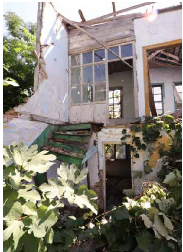
Fig. 3: Interior view of the south wing
