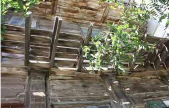
*Fig. 3: Timber projection at the top level of the ground floor on the south façade*
