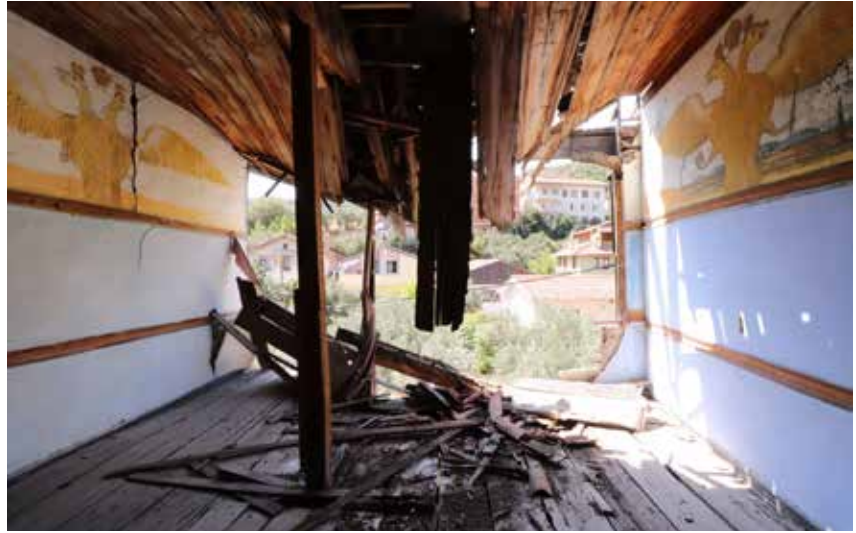
Fig.4: Current condition of the west wall
