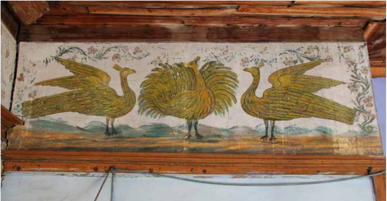
Fig.11: Current condition of the south wall
