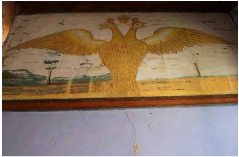
Fig.6: General view of the west wall in the north wing
