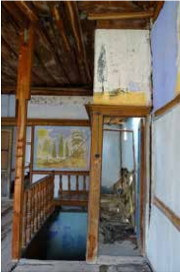
Fig.3: Top of the stairs, facing east
