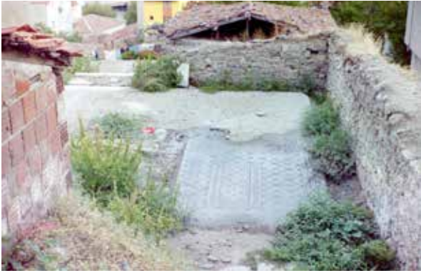
Fig. 6: Tanyeli no.40 Western half of the prayer hall, looking south, terrazzo tiles flooring (1999)
