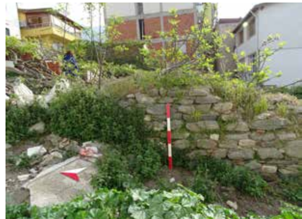
Fig. 2: Western façade detail and sill stone fragment (2019)
