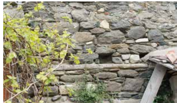
Fig. 3: Timber wall plate in the northern wall and beam holes (2019)
