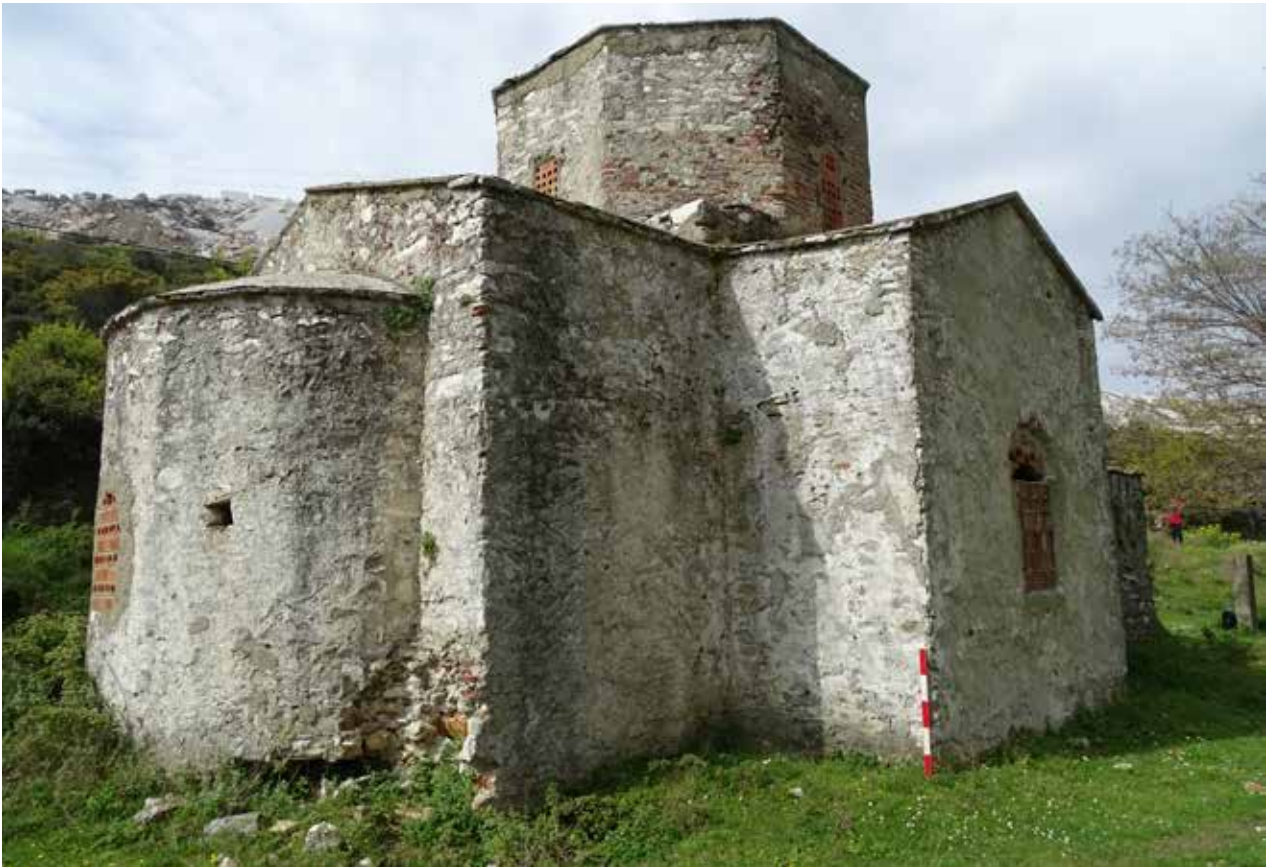
Fig. 2: General view from the northeast
