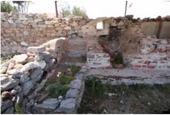
Fig. 10: Stairs and stove
