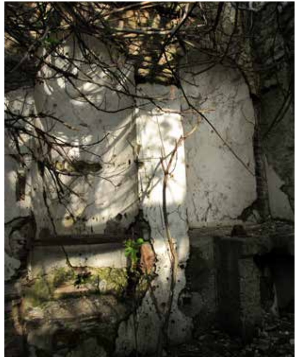
Fig. 4: The niches in the eastern wall of the church
